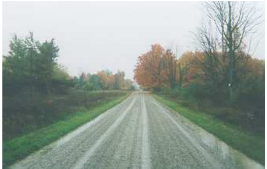
Figure K Typical unpaved county road
