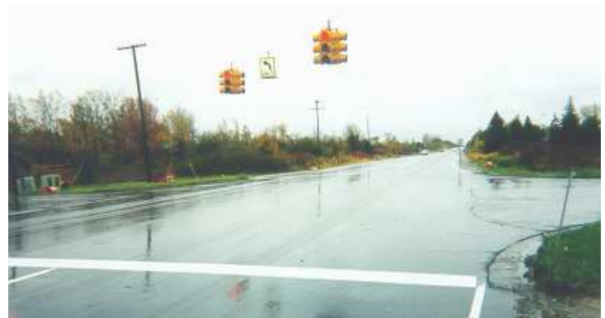
Figure L Typical paved county road
